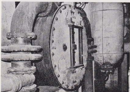
Condensor 2200 kW-turbine
